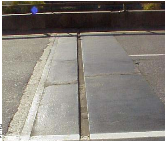
The X.J.S. joint seals gave CDOT a cost-effective, easy installation that is performing well.
