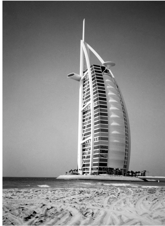
Figure 12. Burj-Al-Arab Hotel, Dubai; a tribute to the use of structural glazing silicone adhesive in a high-rise façade.
